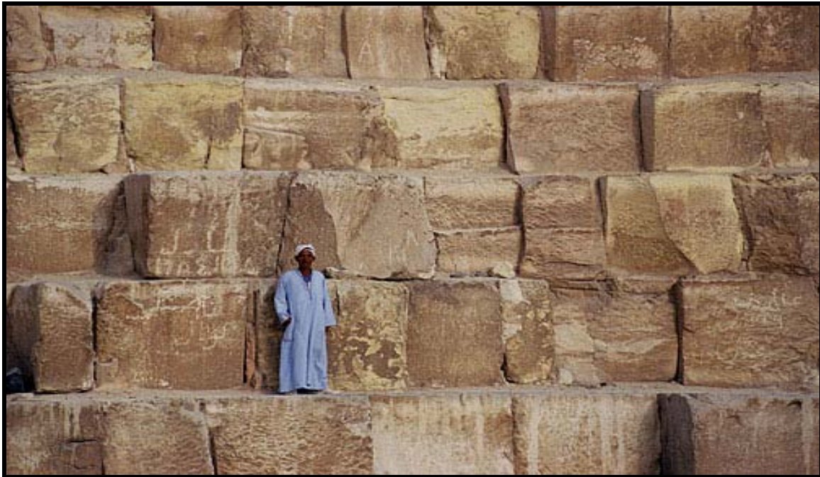
Figure 1.5: Some of the 2,300,000 limestone blocks in the Great pyramid, weighing approximately 15 tonne each. (Courtesy: Martin Gray; sacredsites.com)
